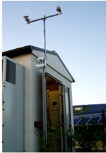
PF2-55 Pole h=2m with brackets for mounting on the wall
