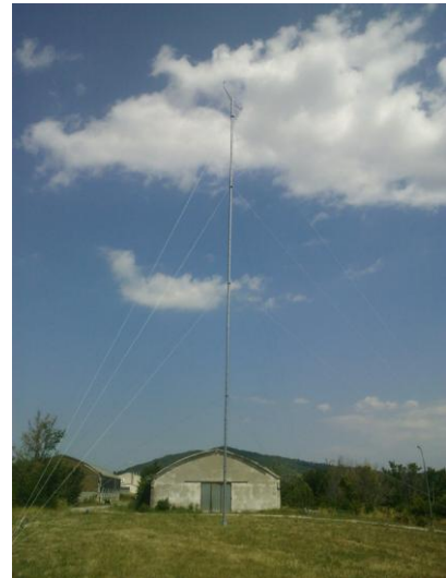
PRF20-60 - Anemometric pole h=20m with guy wires and without civil works
