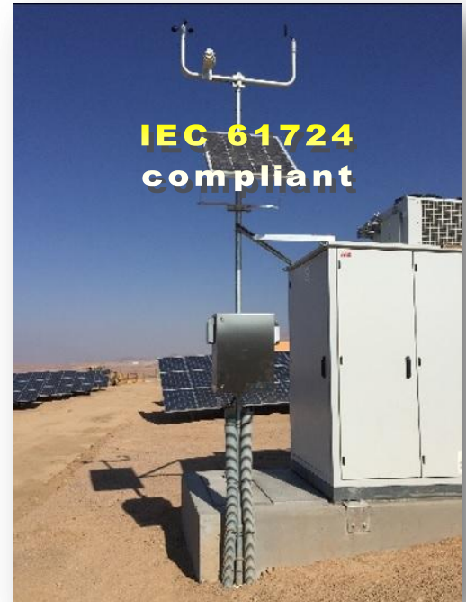
Particular of the meteorological station and of the datalogger enclosure –Jordan installation
