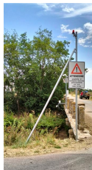
Examples of installation with 3m poles (with webcam, rain gauge and warning lamp)
