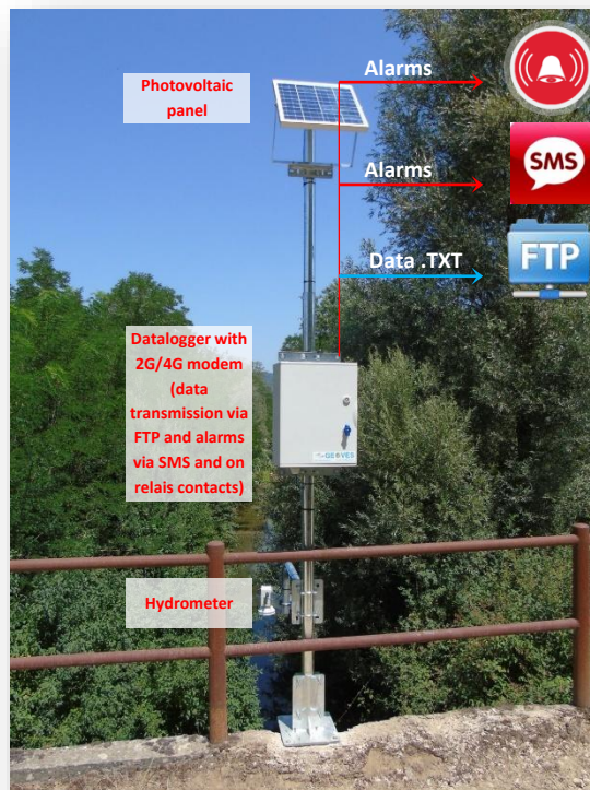
Surface water monitoring and alarm station
